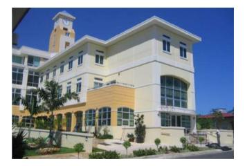
Designed and built by DDD, the project involved the demolition and replacement of an existing facility in order to house the new Student Services and Administration Building for Caribbean University in Bayamon. The project consisted of ground level parking, green areas and a 6 story cast in place concrete structure. In the basement, the facility housed the university's central data center. An additional 4 levels of office and student services space occupied the upper floors.
